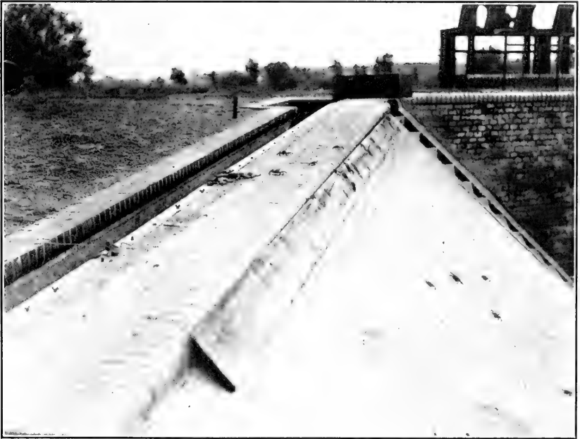
2. Trap projects by the dam in Gruetz on the Havel left wall with trench traps and climbing mitten crabs. (Photographs by Dr. Roehler.)
